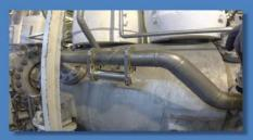
very nign levels of vibration were measured at the balancing pipe of a gas export compressor on an oil and gas installation in the North Sea. Due to thermal expansions, traditional supports could not be applied, and a TVB Damper needed to be retrofitted. After it was mounted on the balancing pipe, 98% of resonating frequencies were dampened and vibration was brought down to an acceptable level.
