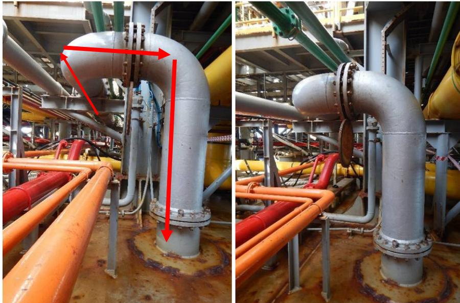
Figure 46 - Branch run down the line to the tank 3C, through a "Figure 8"
