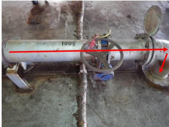
Figure 44 - Branch line to run down the 2C tank, through the BFV-1006
