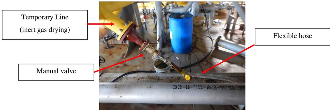
Figure 78 - Connection of submersible pumps with inert gas line
