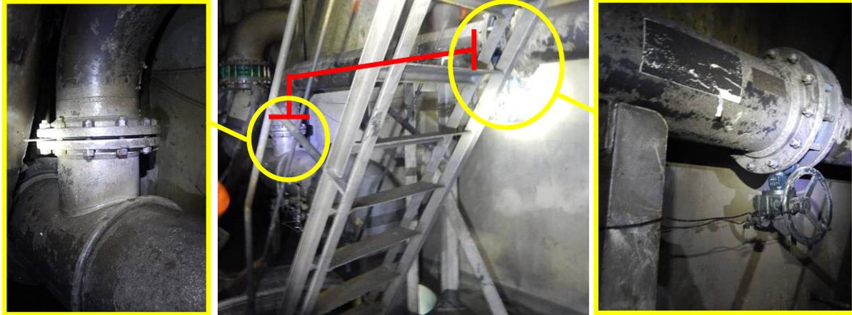
Figure 124 - Excerpt pipe installed between the spade and BFV-1005 valve
