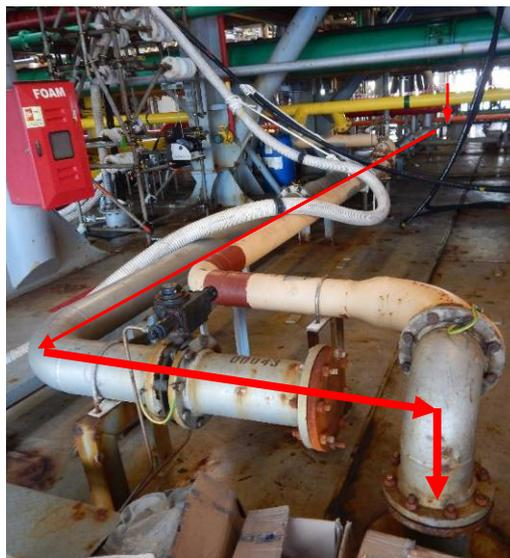
Figure 47 - Gangway line to the starboard header past the OD-043
