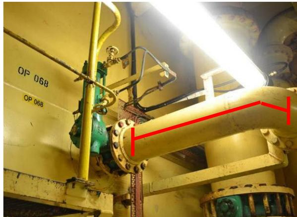
Figure 125 - Excerpt pipe installed between spade and OP-068 valve<sup>201</sup>
