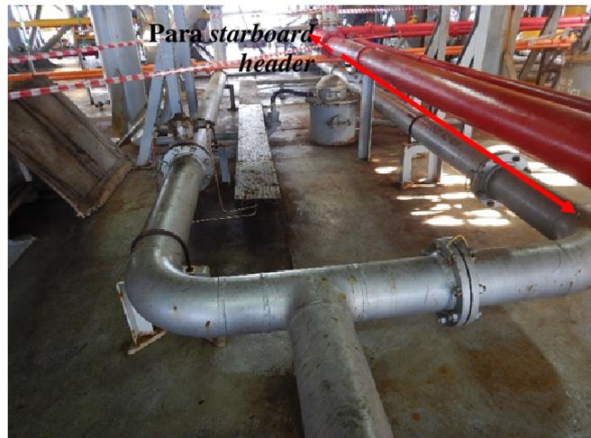
Figure 43 – Run down division through the line to the tank 2C, 3C tank and the starboard header
