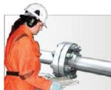
3. Verify that all the bolts are tightened with the right moment. See the tightening procedure.
